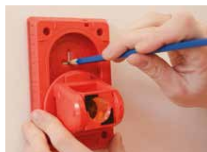
Slide the prism to one side and mark the target position with a pencil.
