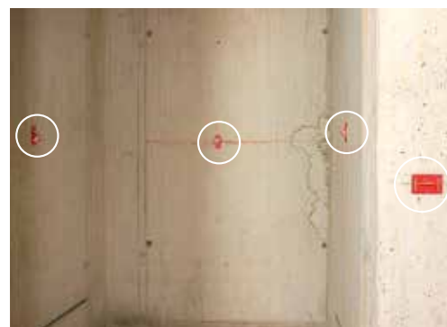
RS21 and RS21: perfect reference points for FFL and axes in the area of elevator shafts
