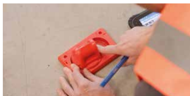
Slide the prism to one side and mark the target position with a pencil.
